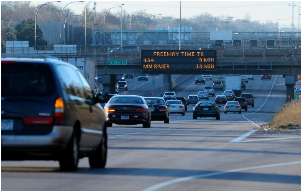
Figure 3: Dynamic Message Sign on Interstate 35W South
