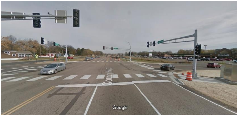
Figure 6. An example of an intersection with incomplete pedestrian facilities 20
