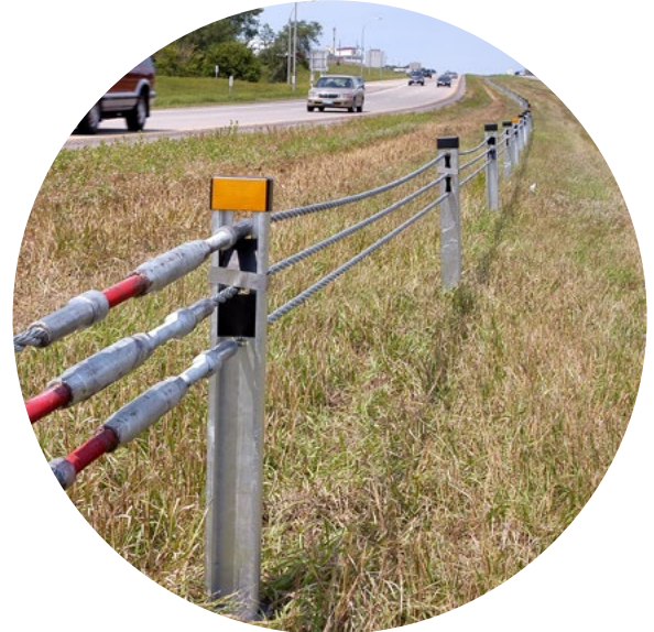
Cable Median Barriers are one example of a traveler safety feature.
