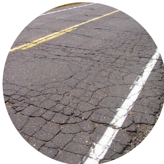
Example of a road in poor condition. This pavement would receive a low RQI based on its degree of cracking and smoothness of ride.
